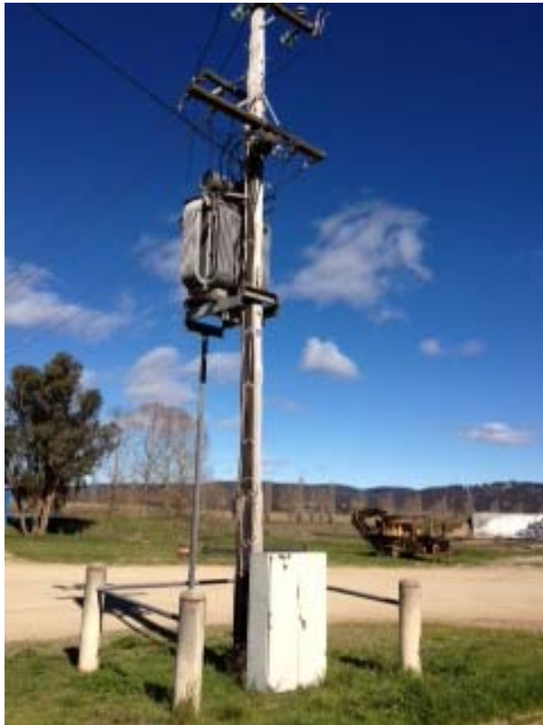
FIGURE 6: MAIN TRANSFORMER POLE AND POWER SWITCH (INSERT)
